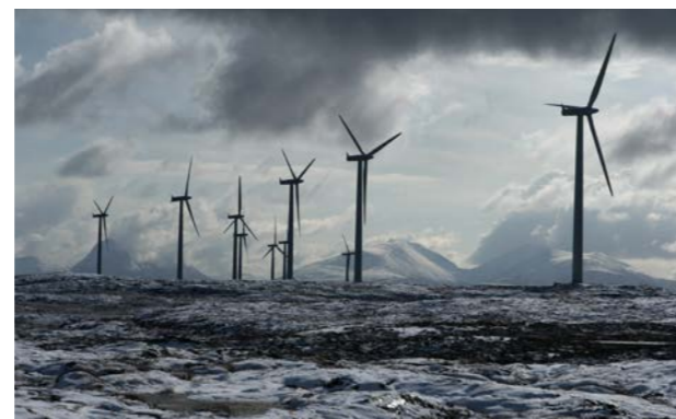
Smøla Wind Farm. Photo: Statkraft / flickr
